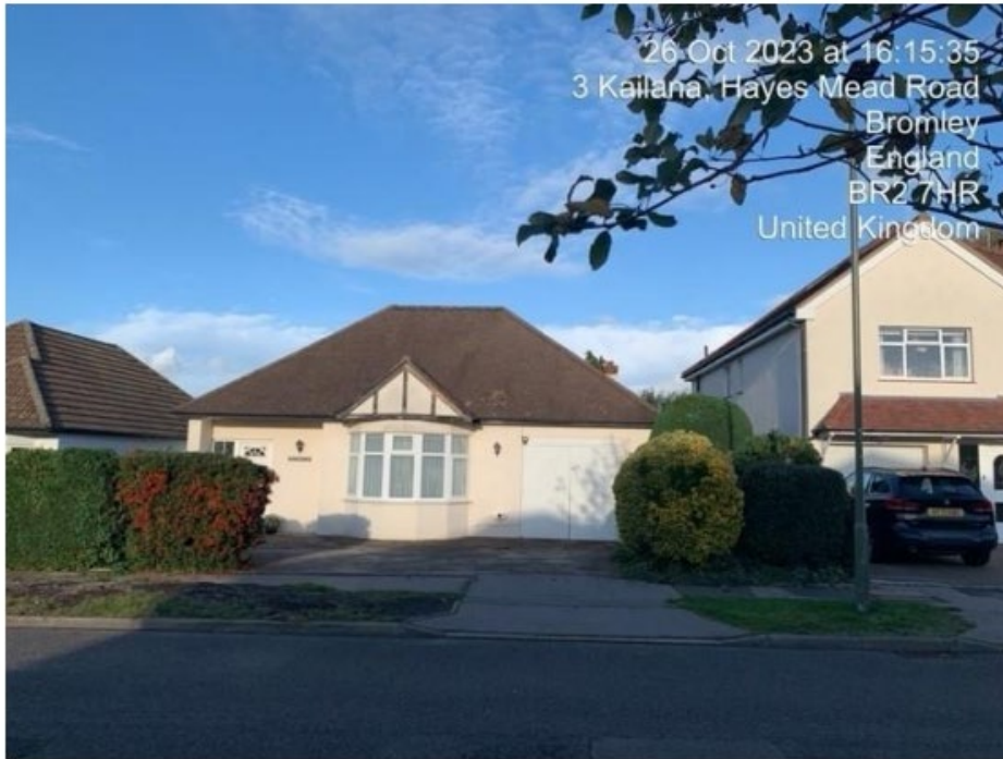
Figure 3 – photo of the site viewing from Hayes Mead Road
